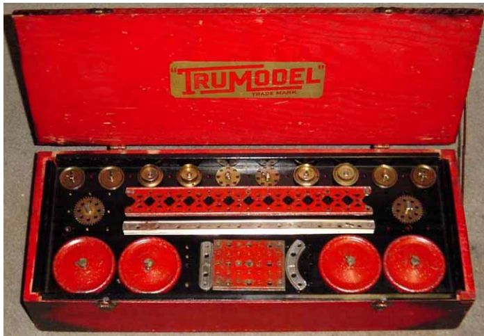
1929 #77 TruModel set. The Wholesaler sets were similar to the Gilbert line, but contained some unique parts. The girders had just holes in them instead of a truss pattern. Most of the same models were pictured in the manuals but the drawings were updated to show the different parts.
